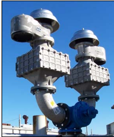
Figure 6-1. Redundant PRV assembly
