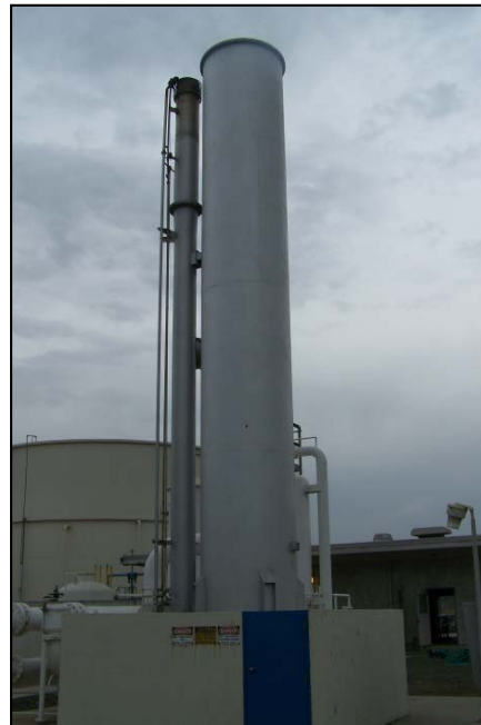
Figure 3-14. Newer waste gas flares at the WPCP
