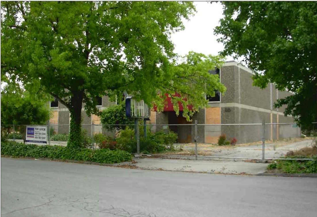
Photo 2 - One of two existing two-story buildings on the project site. The vacant building fronts East Rosemary Street on the east half of the site. The photo was taken from East Rosemary Street looking south.
