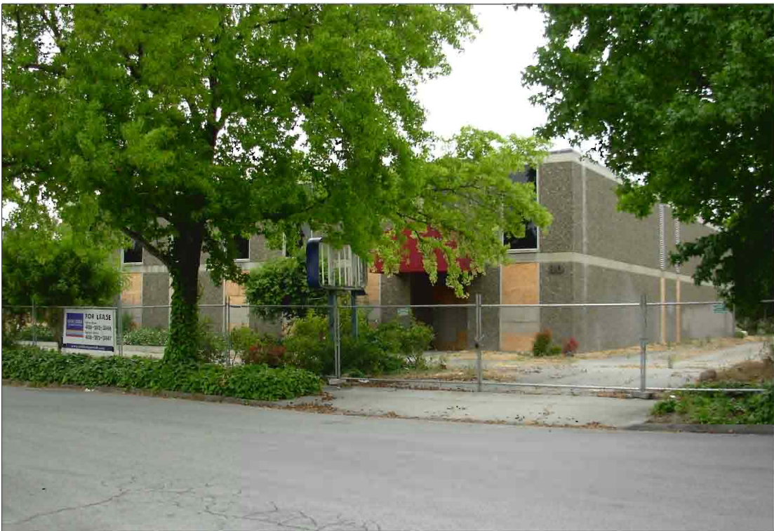
Photo 2 - One of two existing two-story buildings on the project site. The vacant building fronts East Rosemary Street on the east half of the site. The photo was taken from East Rosemary Street looking south.
