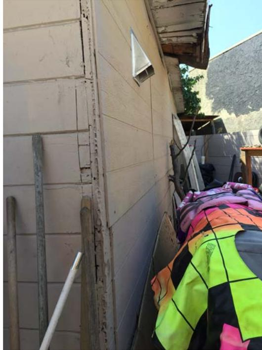
Photograph 4. View southeast of southwest elevation. Note the original wood board cladding and replacement.
