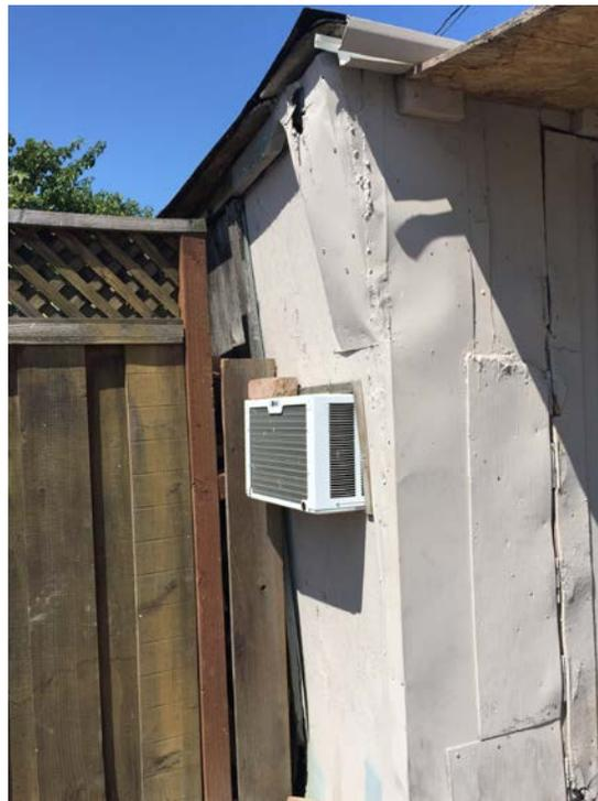
Photograph 5. View west of southeast and northeast elevations. Note the replacement aluminum and plywood siding.
