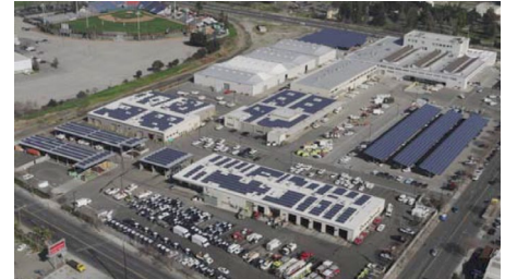
Photo: DRI Energy installation of 1.24 MW at the City of San José Central Service Yard.
