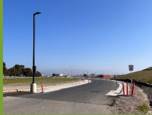
Newly paved roadway
