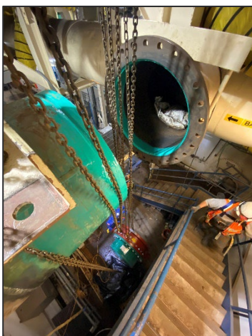
Lifting valve into place as part of Filter Rehabilitation project
