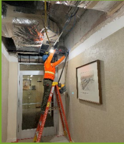
Upgrading fire system within Admin Building
