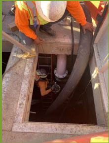
Confined space work
