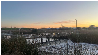
New Weir, bridge lights, and rip rap
