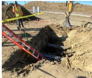
Initial site prep excavation work
