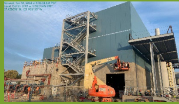
Dewatering Building south staircase and enclosure under construction
