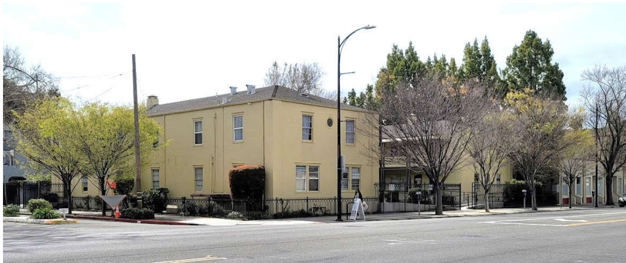
Photograph 3 610-650 E. Santa Clara Street View: East corner showing the front and east facades Date and Camera orientation: March 14, 2021 Facing-Southwest
