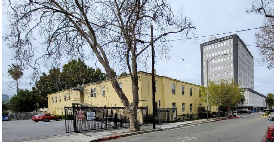
Photograph 4 610-650 E. Santa Clara Street View: Southeast corner, showing the rear and east facades Date and Camera orientation: March 14, 2021 Facing-Northwest
