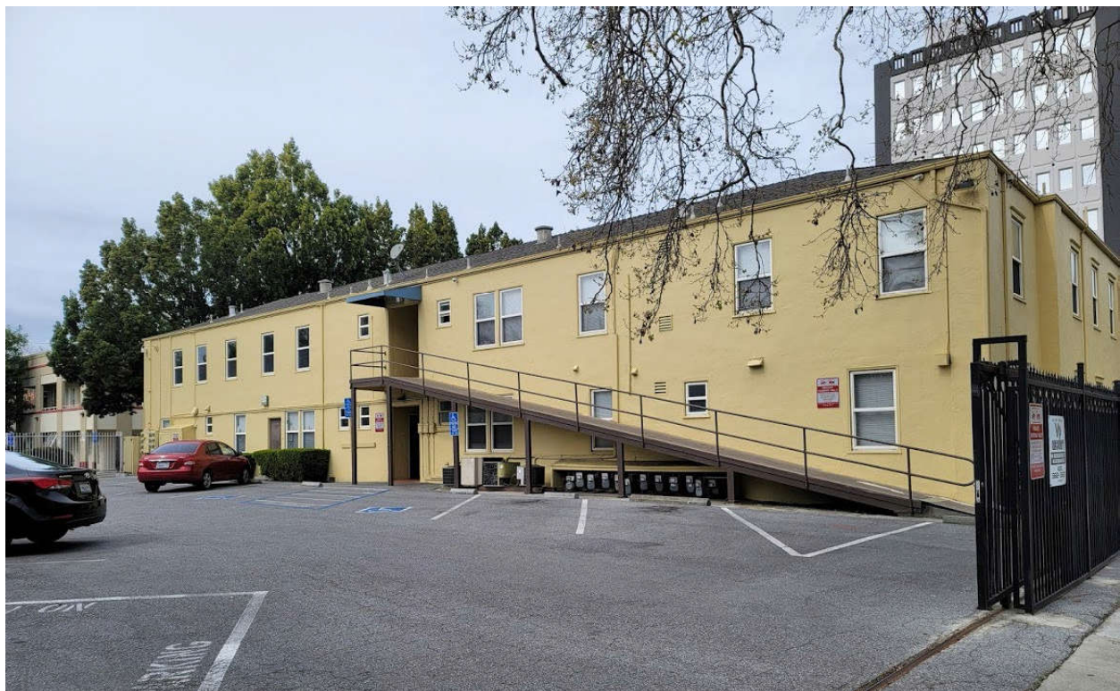
Photograph 5 610-650E. Santa Clara Street View: Rear (South) Façade with ramp Date and Camera orientation: March 14, 2021 Facing-North
