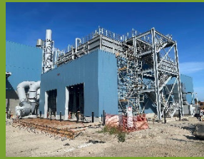
Truck loadout building approaching construction completion
