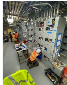
Master Control Center AF2 Installation Work
