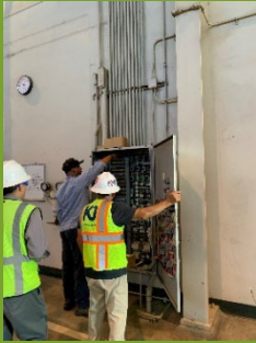
Upgrading fire system within Building 40
