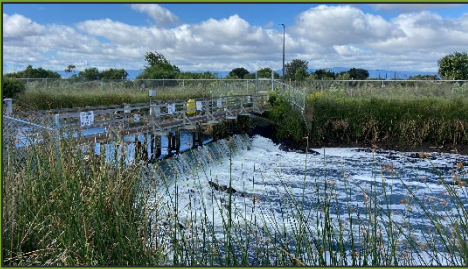
Newly improved outfall bridge with new weir, bridge lights and riprap
