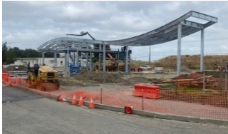
Initial site prep excavation work
