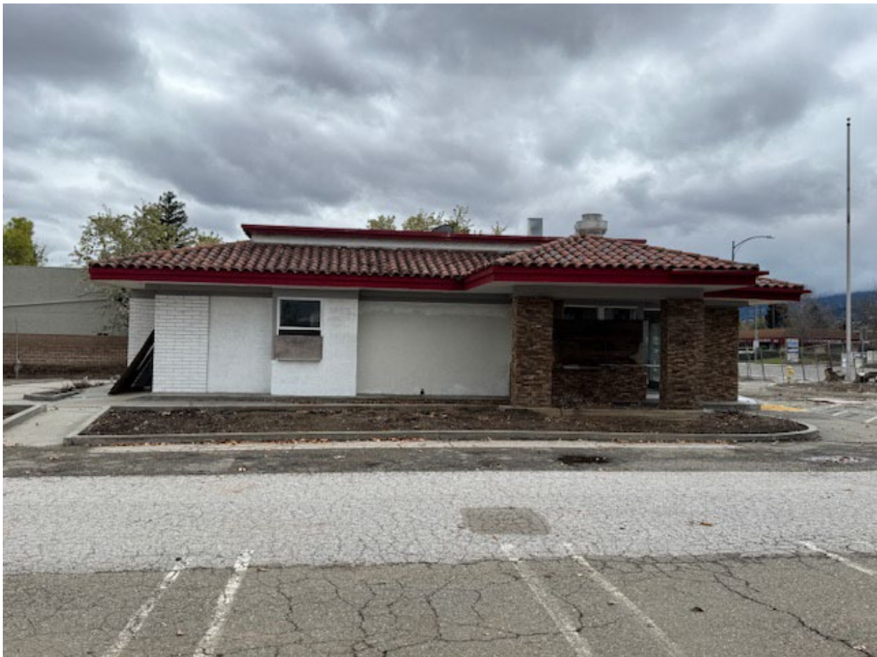
Photograph 2 100 De Anza Blvd. San Jose View: north façade with drive-through canopy.
