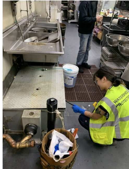
FIGURE 3. ENVIRONMENTAL INSPECTOR OPENING A GREASE TRAP
