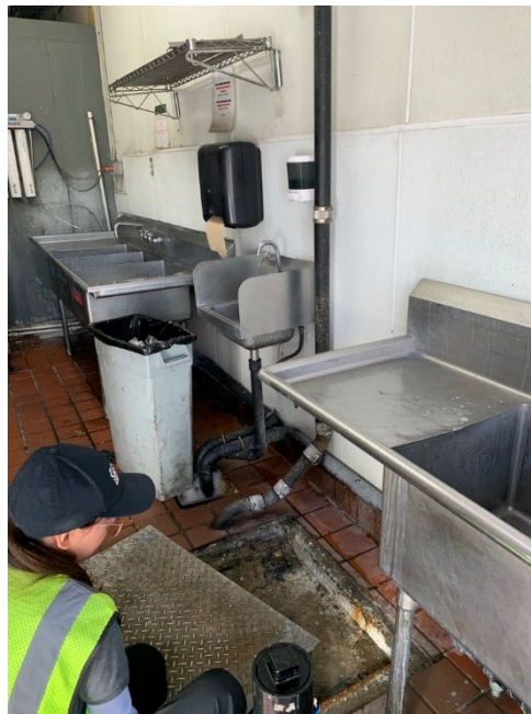
FIGURE 3. ENVIRONMENTAL INSPECTOR OPENING A GREASE TRAP
