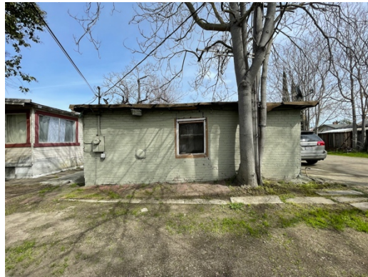
Figure 15. Southwest elevation, accessory dwelling unit.
