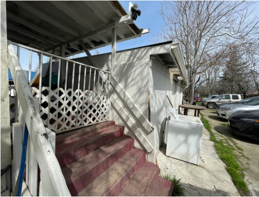
Figure 12. Southwest elevation, plywood storage building.
