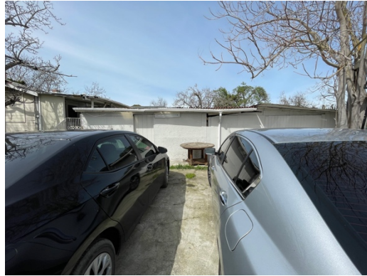
Figure 13. Southeast elevation, plywood storage building.
