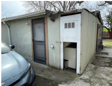
Figure 17. Northeast elevation, accessory dwelling unit.
