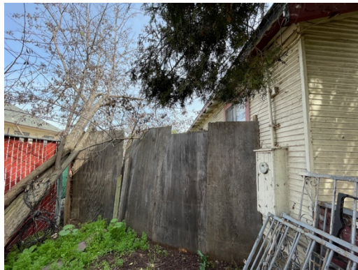
Figure 6. Northwest side elevation behind plywood barrier.
