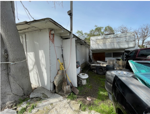
Figure 14. Northeast elevation, plywood storage building.
