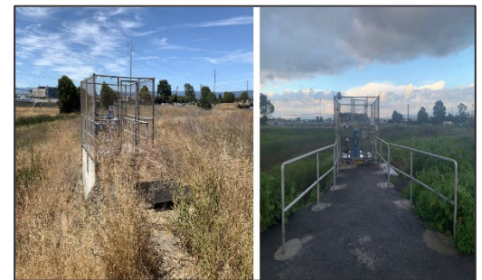
Before and after pictures of the rehabilitated Legacy Lagoon Pump Station
