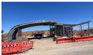
Steel frame nearing completion
