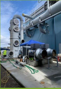
Odor equipment installation
