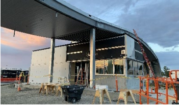
Steel frame and guard house construction
