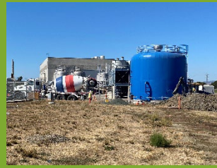
Newly painted and coated water tank.
