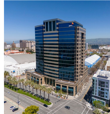
Sobrato Tower 488 Almaden Blvd (2002)
