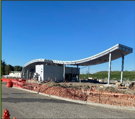
RWF Main Entrance Improvements project under construction
