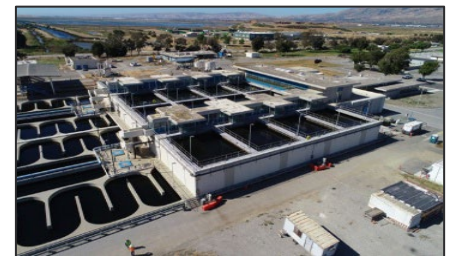
The Filter Rehabilitation project area includes the filtration tanks, walkways, filtration building, and filtration influent pump station (FIPS)
