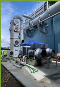
Odor equipment installation
