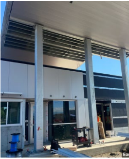
Development of guardhouse improvements.
