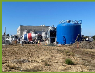
Newly painted and coated water tank.
