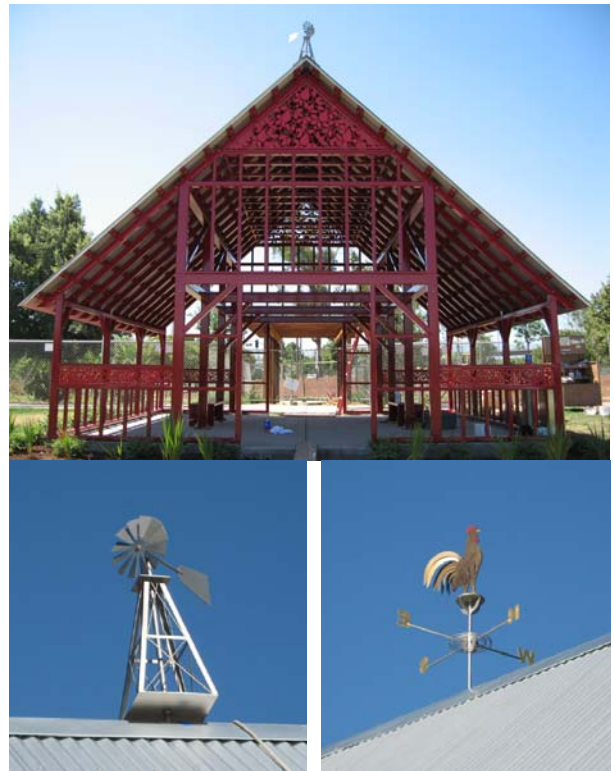
Above: View of The Last Barn during the final stages of construction and details of the roof vanes and filigree work.
