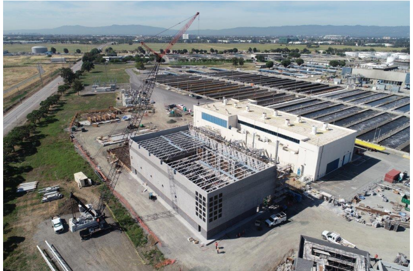
Figure 1: Cogeneration Main Generator Building roof truss installation
