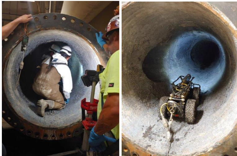
Figure 4: Manned entry and CCTV process piping inspection
