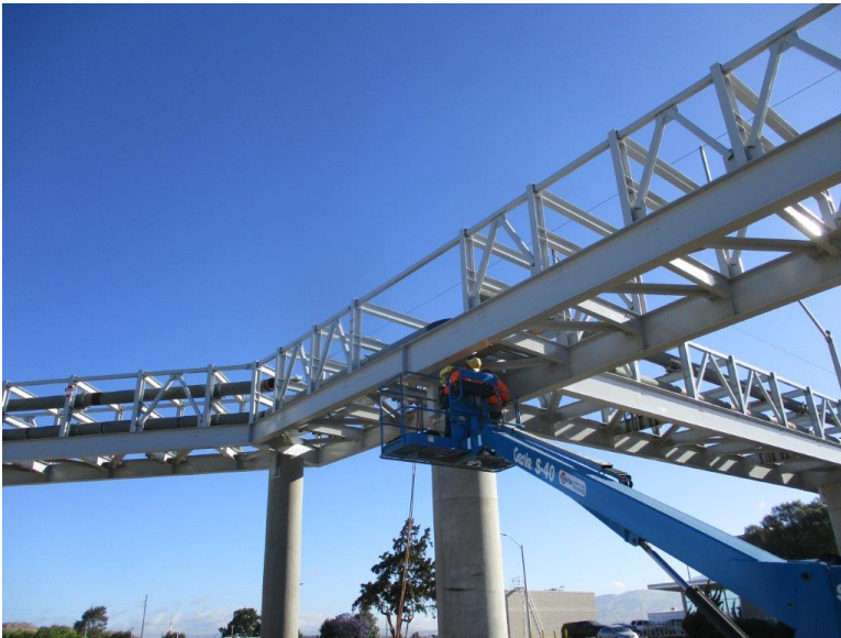
Figure 5: Elevated Pipe Rack Installation
