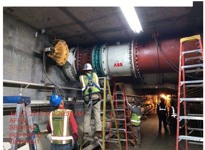
Figure 5: Contractor tightening bolts on new meter and pipes
