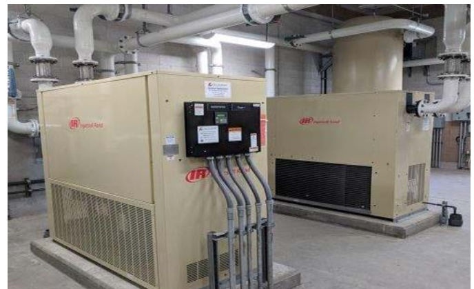
Figure 9: Refrigerated Air Driers
