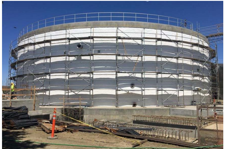
Figure 1: Recently applied insulation on Digester 5
