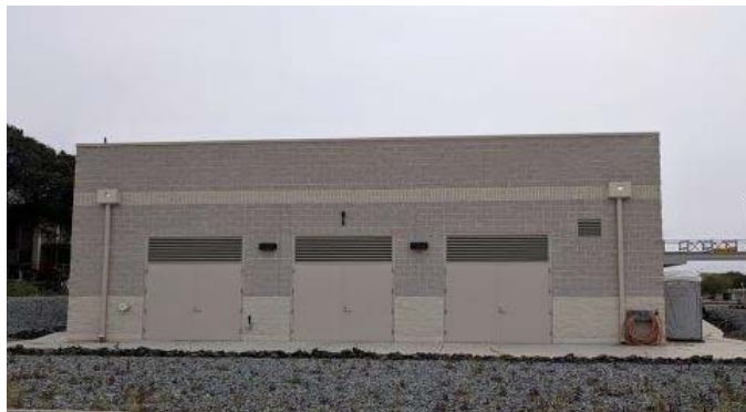
Figure 8: New Plant Air Compressor Building
