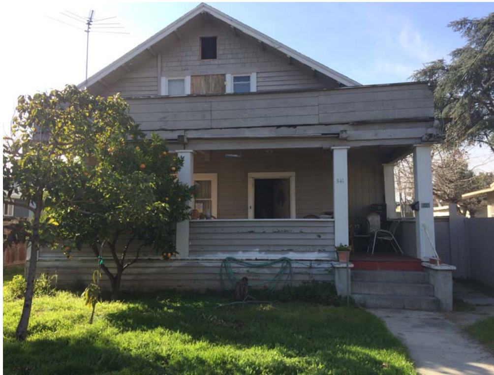
Photo 1: Front of Subject Property (East).
