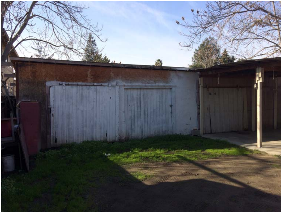
Photo 4: Storage unit West part of Subject Property.
