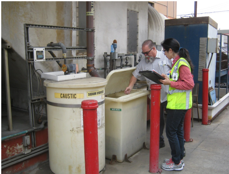
FIGURE 3. A SOURCE CONTROL TEAM MEMBER PERFORMING A SITE INSPECTION
