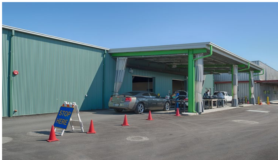
FIGURE 5. HHW FACILITY AT THE SJ EIC.
