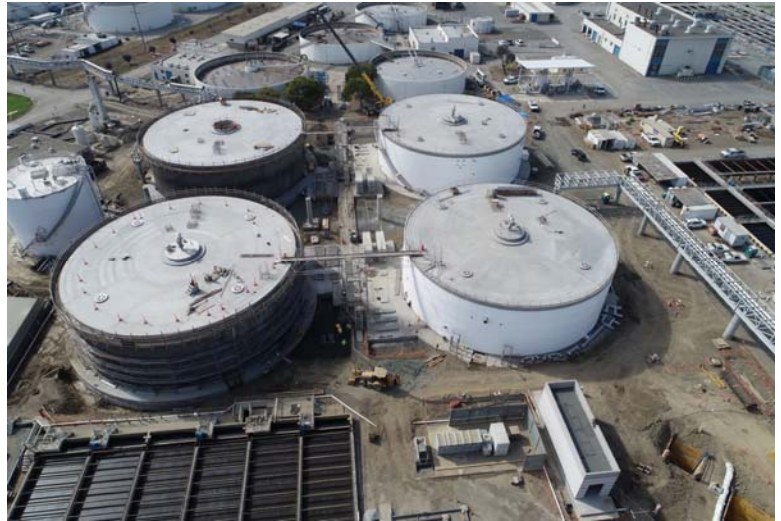
Figure 1: Completed exterior insulation on Digesters 5 & 6
