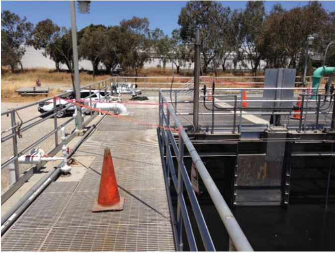
Figure 4: Area cordoned off at the Emergency Basin Overflow Structure to protect a nesting mourning dove
