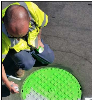
A member of DOT marks a manhole electric green.
