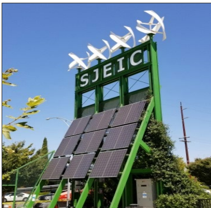
FIGURE 5. SJ EIC, LOCATION OF ONE OF SANTA CLARA'S HHW FACILITIES
